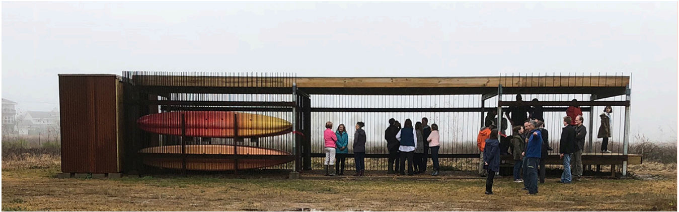
Figure 1. STORE provides shaded teaching space and storage for Artist Boat’s educational programs. Image credit: Gulf Coast DesignLab.
